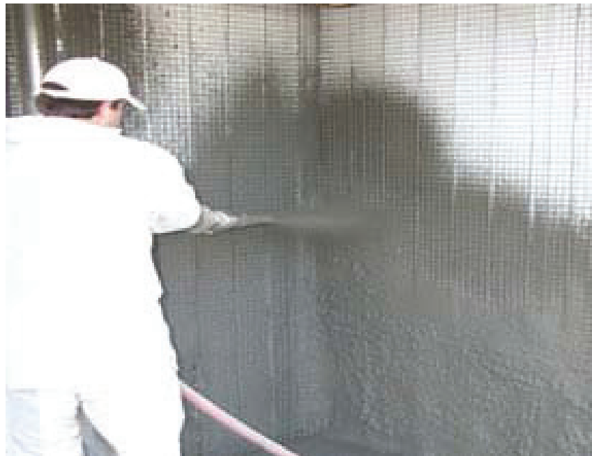
Figure 5 — SCIP system being covered with shotcrete.
